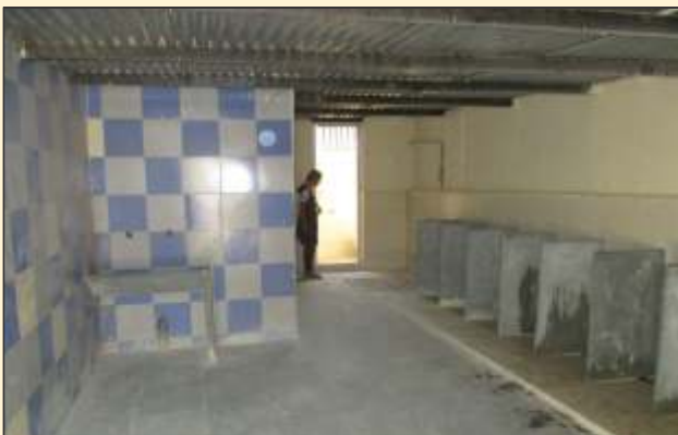
New toilet constructed by RC Kalol
